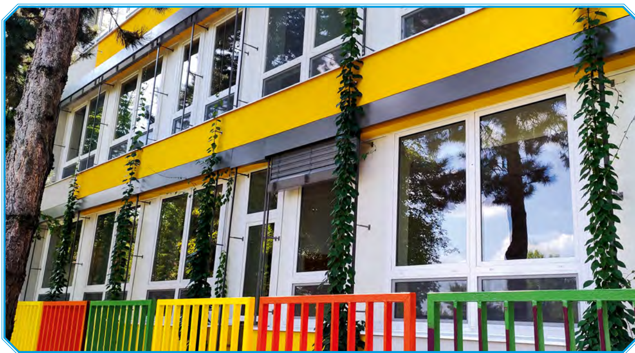
Picture No.15: Kindergarden Kolískova: Three vegetated walls made of stainless steel mesh with climbing plants and fifteen vertical wire systems with wrapping plants (source: archive of the Bratislava-Karlova Ves Municipality)
