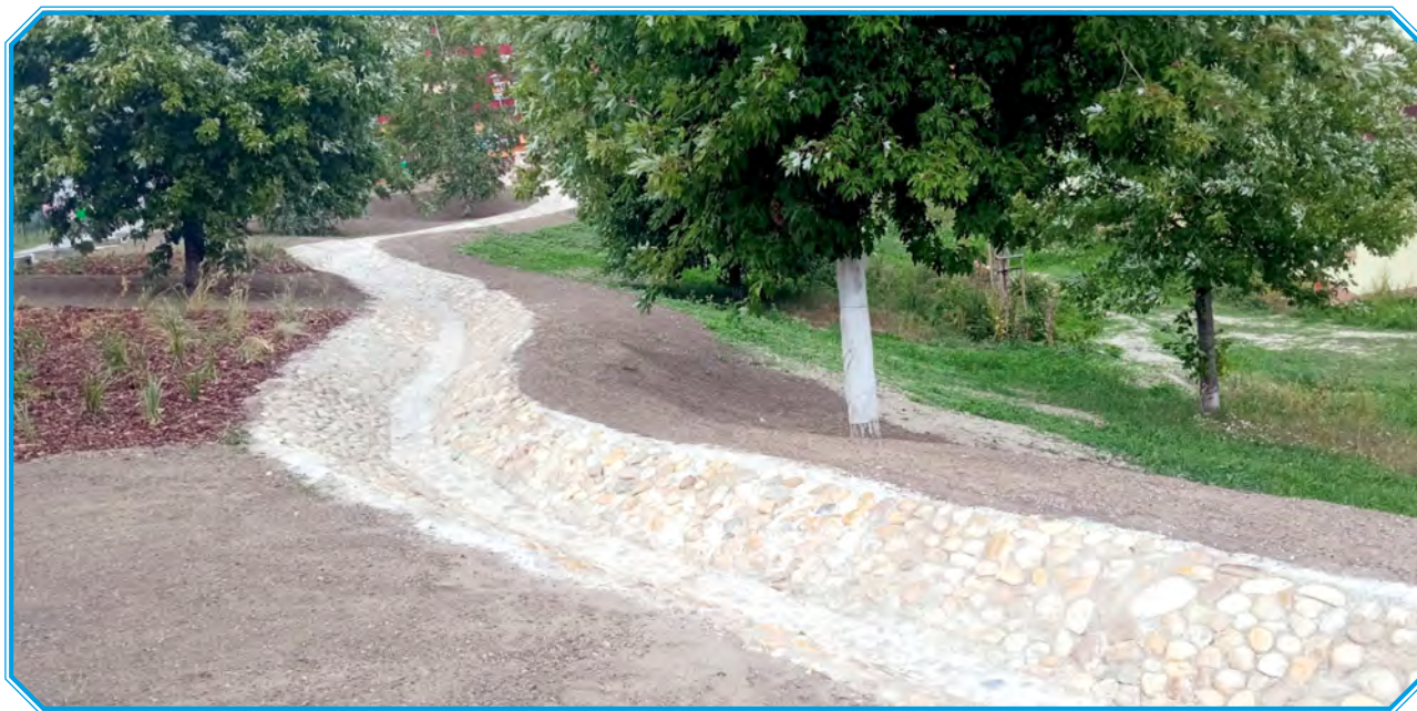
Picture No. 26: Phase 3 – construction of a artificial stream using retained rainwater (source: archive of the Municipality of Bratislava-Karlova Ves)
