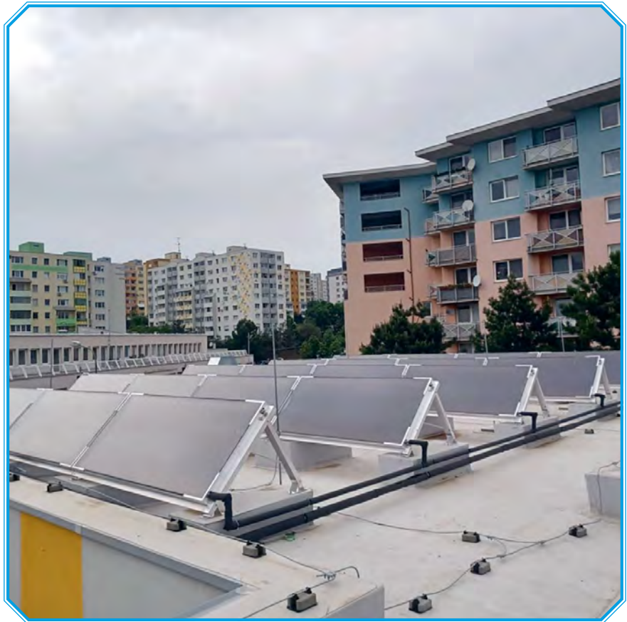
Picture No. 18 and No. 19: Hot water tanks heated through photovoltaic panels (source: archive of the Municipality of Bratislava-Karlova Ves)
