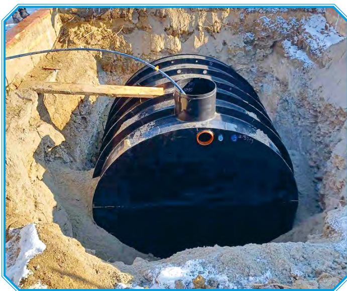
Picture No.17: Underground retention tank for rainwater (source: archives of Bratislava-Karlova Ves Municipality)
