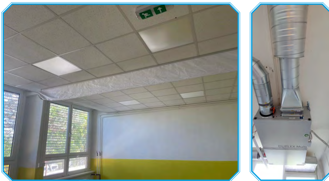
Picture No.13: Controlled ventilation with heat recovery – fabric sleeves under the ceiling with fresh air supply. Pipes that draw in fresh air from atria and exhaust waste air. (source: archive of Bratislava-Karlova Ves Municipality)
