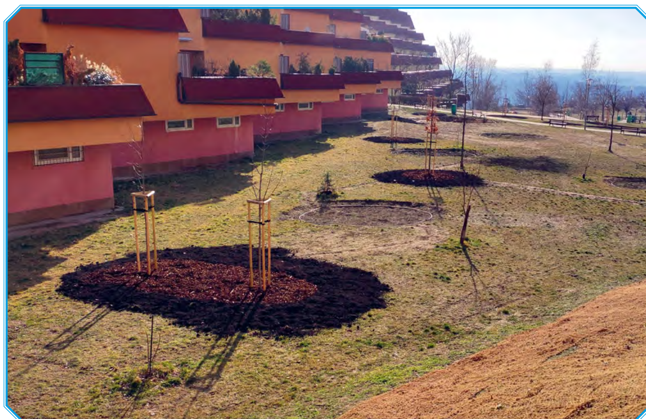
Picture No. 21: Terrain modeling, tree planting with irrigation from captured water, retention bowl areas with planted meadow mix (source: archive of the Municipality of Bratislava-Karlova Ves)
