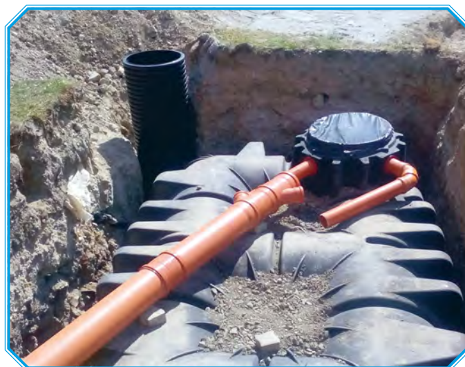
Picture No. 23: Underground retention tanks for rainwater capturing (source: archive of the Municipality of Bratislava-Karlova Ves)
