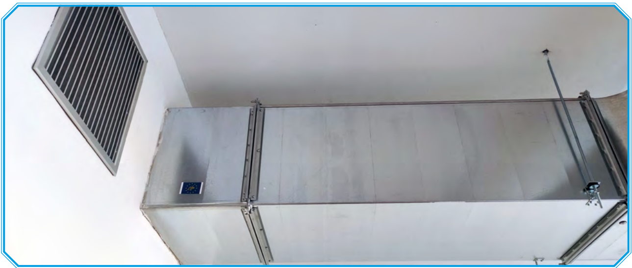
Picture No. 32 and 33: Controlled ventilation with heat recovery in classrooms, bedrooms and in the kitchen (source: archive of the Municipality of Bratislava-Karlova Ves)
