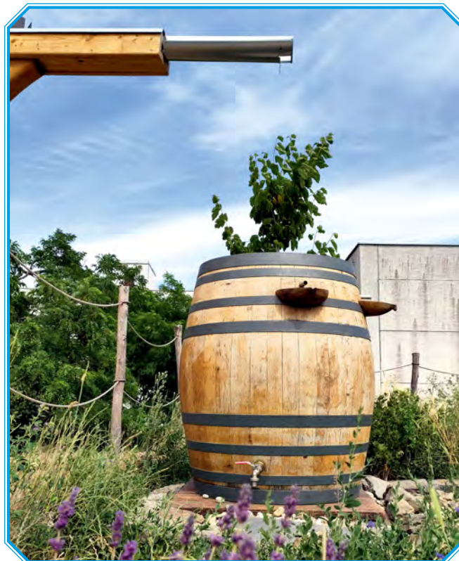
Picture No. 4: Gazebo for the needs of an outdoor eco-classroom near the school garden in the sports and recreation area Majerníkova 60-62, Bratislava-Karlova Ves Municipality. Capturing rainwater from the gazebo roof in a tank and utilizing it to irrigate fruit bushes and herbs was a part of eco-educational activities. The overflow from the tank at the top provides drinking water for birds and insects. (source: archives of the Municipality of Bratislava-Karlova Ves)
