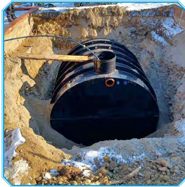
Picture No. 36: Underground retention tank for rainwater collection in kindergarten ground (source: archive of the Bratislava-Karlova Ves Municipality)
